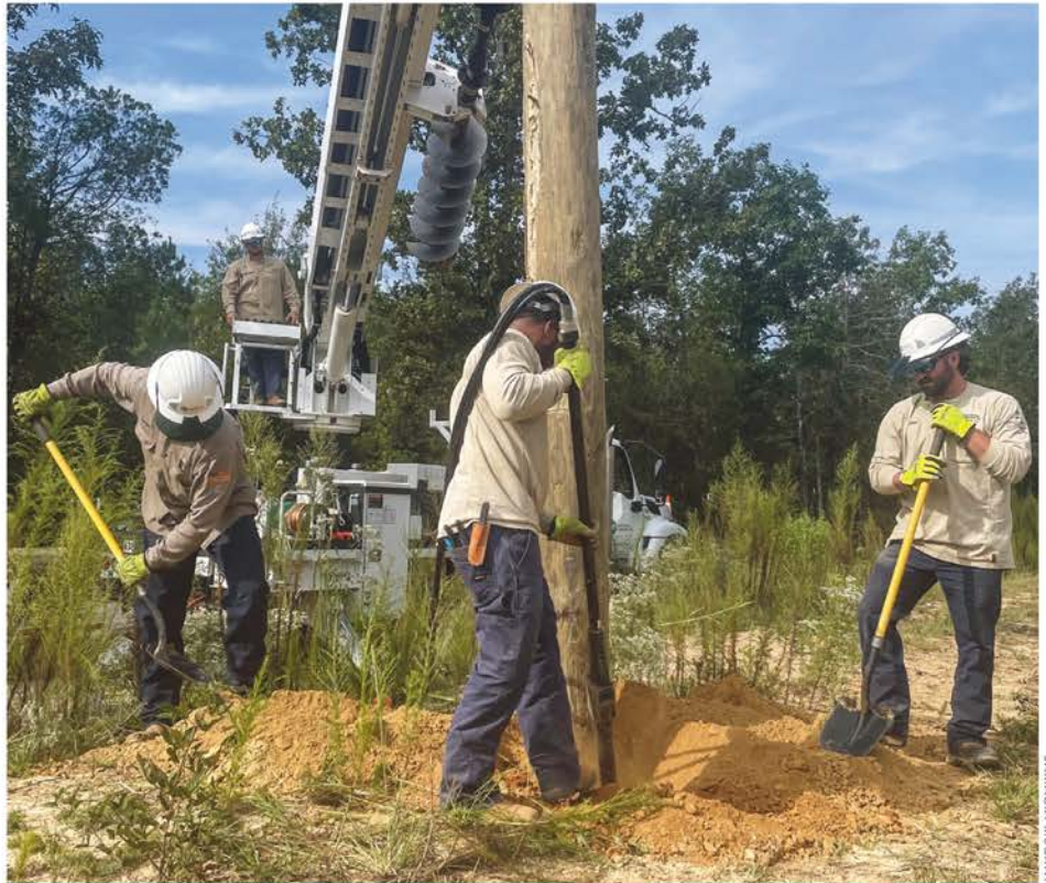
Severe storms often damage or break power poles. The replacement process requires a crew of four lineworkers approximately four hours to complete.
