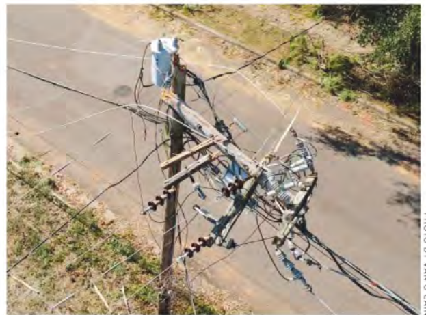
Hurricane Helene's powerful winds broke utility poles like matchsticks. The storm's destruction resulted in the replacement of 1,500 poles on Aiken Electric's system.
